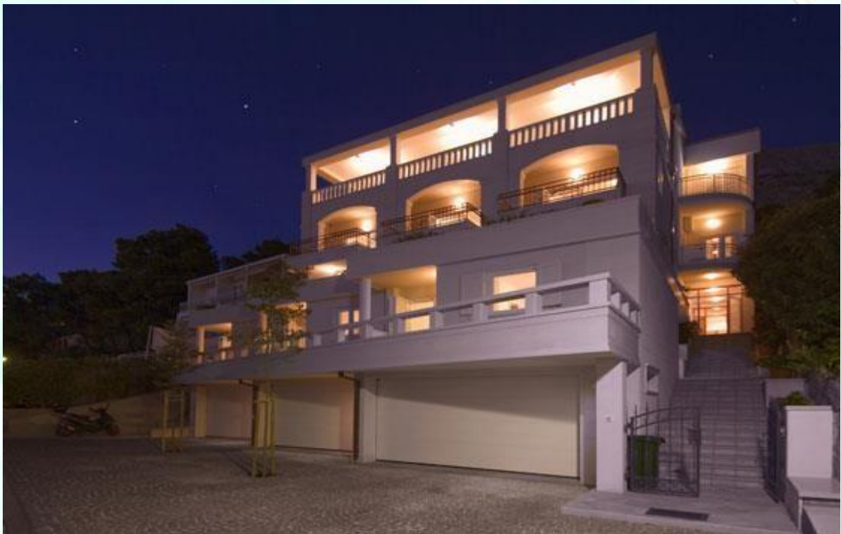
This apartment is located on the upper ground floor (first row of balconies)
